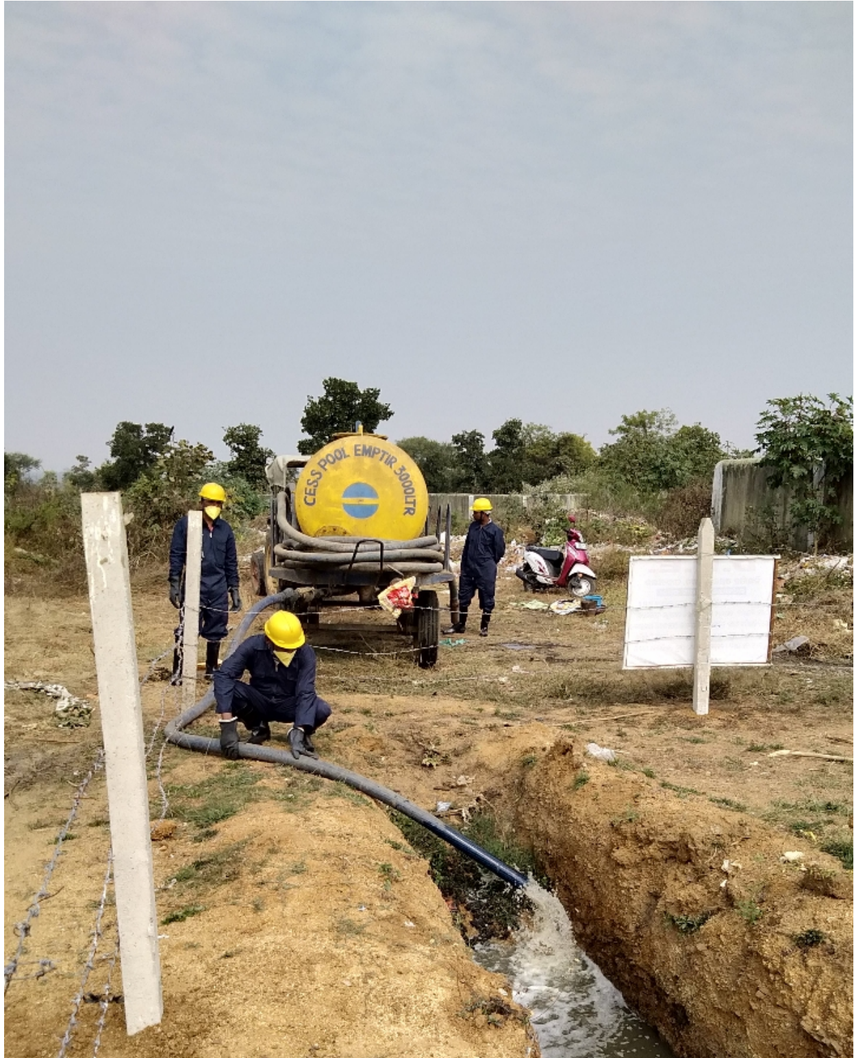
Image 1: DRE trench operation in Odisha Source: TSU-PMU EY Odisha
